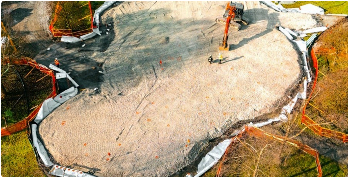
Aerial view: ~646 m³ of Enviro-Rock placed across the playground footprint.
